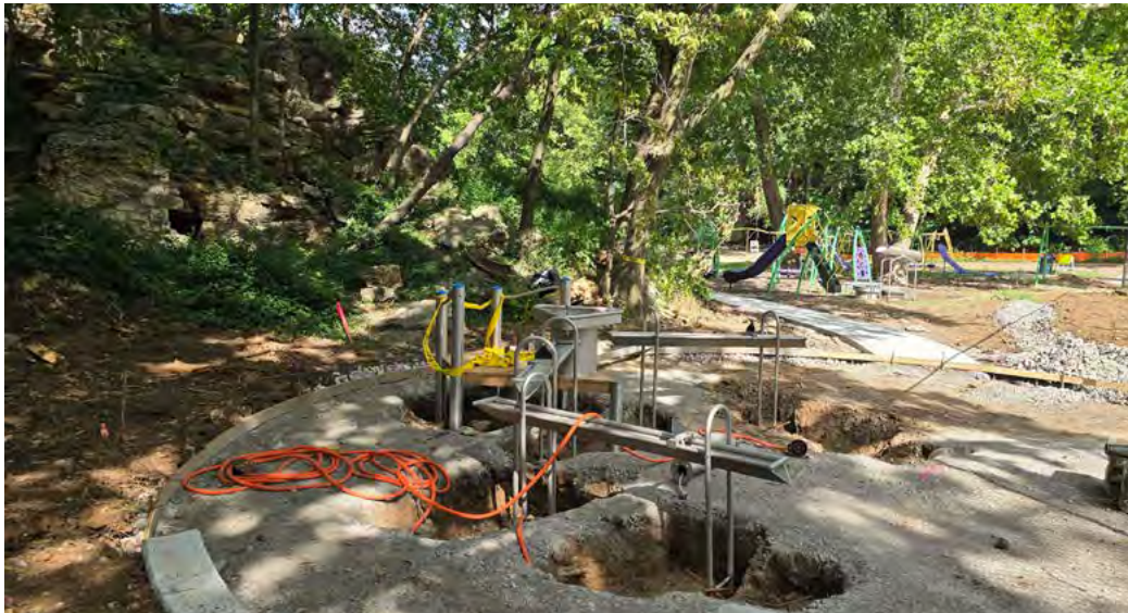
Water Play On-Going Construction
