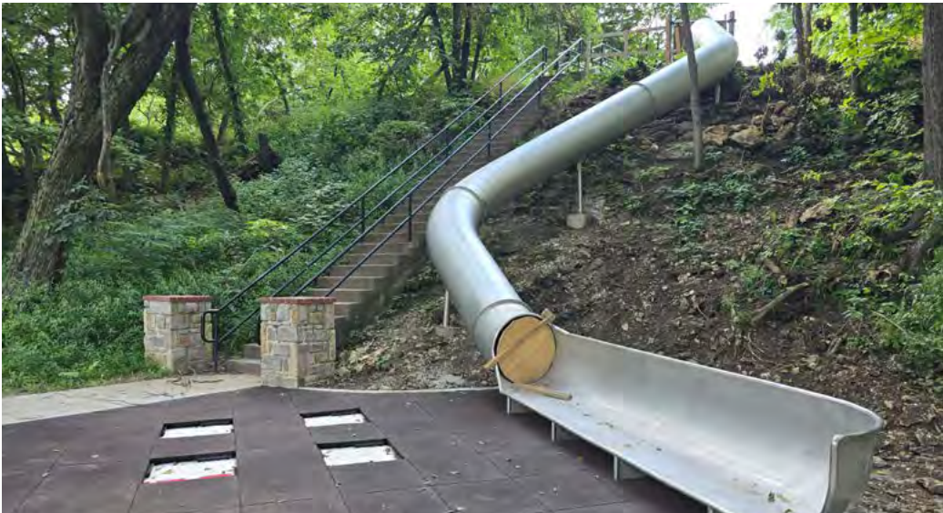
Slide On-Going Construction
