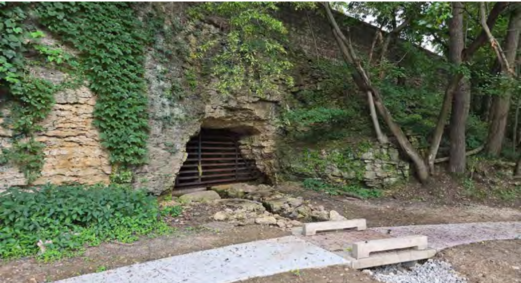
Cave On-Going Construction
